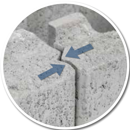
Interlocking tongue and groove joints
