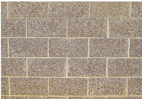
Figure 2 Typical block wall after laying (b)
