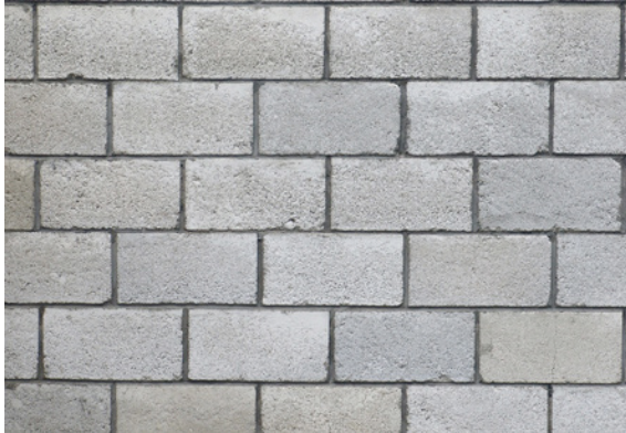
Figure 1 Typical block wall after laying (a)
