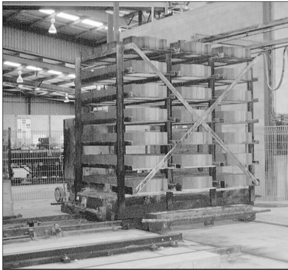
Figure 17 Automatic Rack-transfer Car System, Handling Loaded Racks to and from Curing Chambers
